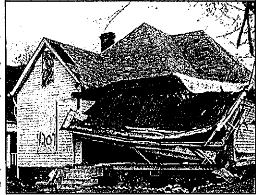
Damage in East End Conservation Zone of Nashville following the April 1998 tornado. Source: Phil Thomason
