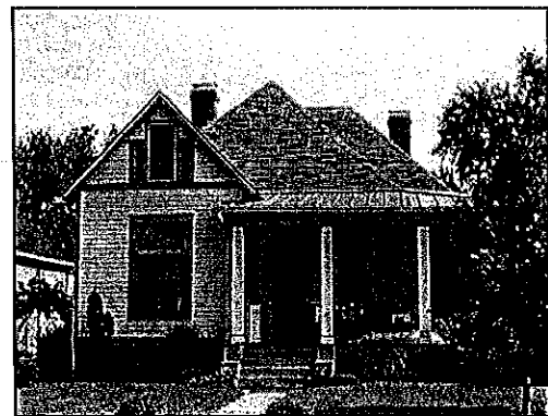
Repairs in East End Conservation Zone of Nashville following the April 1998 tornado. Source: Phil Thomason
