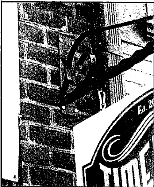
Require fastening methods that do not damage the building. Fasteners should go in mortar joints NOT bricks as shown above. NAPC file photo
