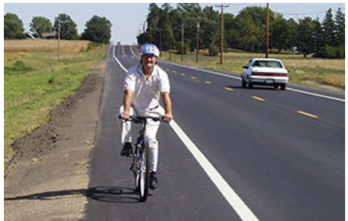
Photo 9.5: Paved shoulder along roadway
