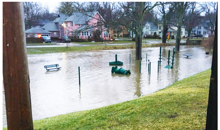
Pictured: Lee Austin Park serving as stormwater storage area.
